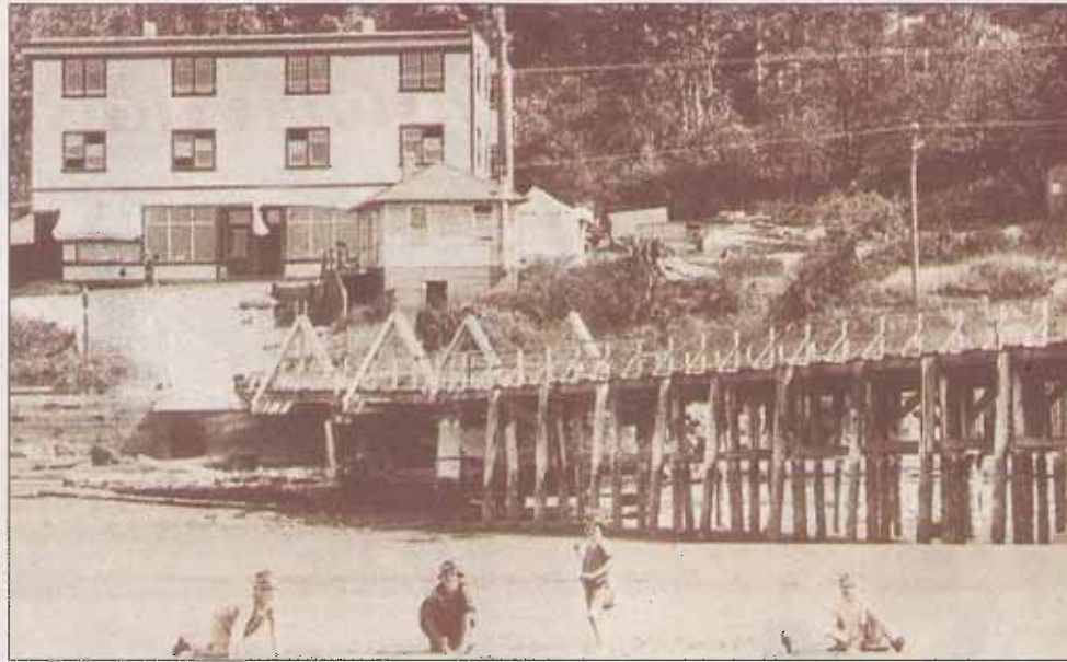
At various times from the 1920s to the '70s, the building at the foot of the pier (above) served as police station, jail, library, Chamber of Commerce office, and washrooms. Above right, the public washrooms in 1980; below, washrooms at West Beach are torn down last year.
